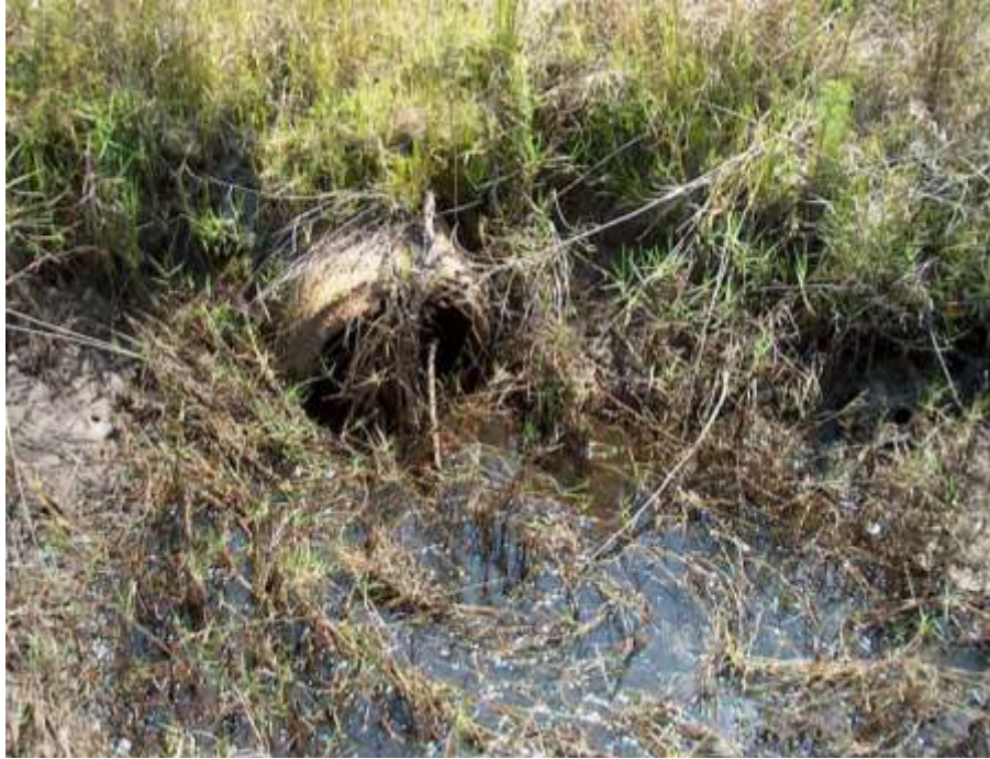
Figure 7 Outfall pipe at Botheration Bayou in West Bay. Bay County, Florida
